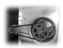
Figure 16: 6 to 20-ton blower motor and fan belt assembly.
